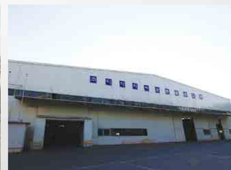
SIC / Cold Forging Plant
