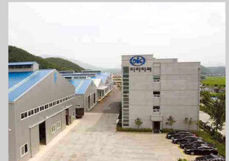
사무동/ Office Building
